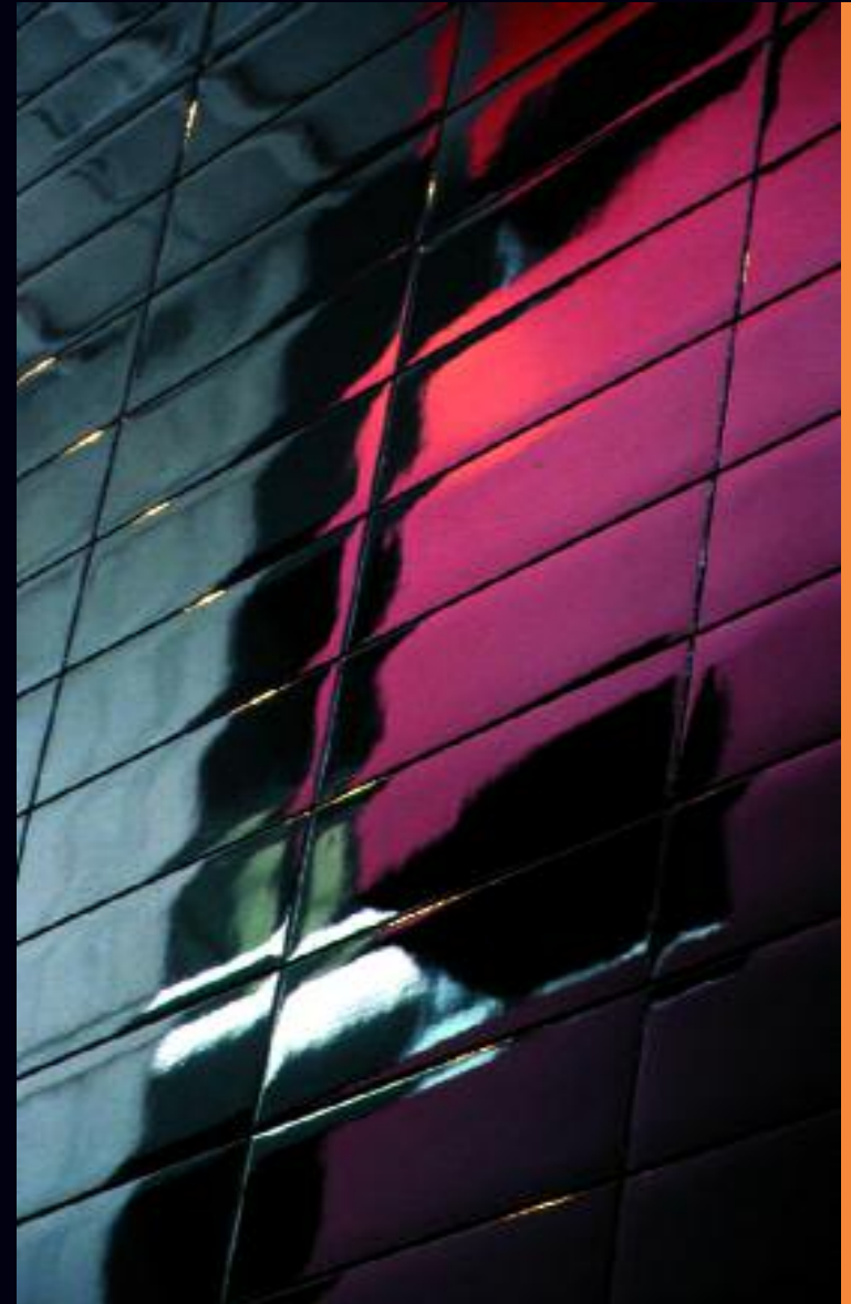
The shiny glazed porcelain panels produced by Vitra reflect the sun on the façade, and surround the boxes on the inner street, so forming an interior element
